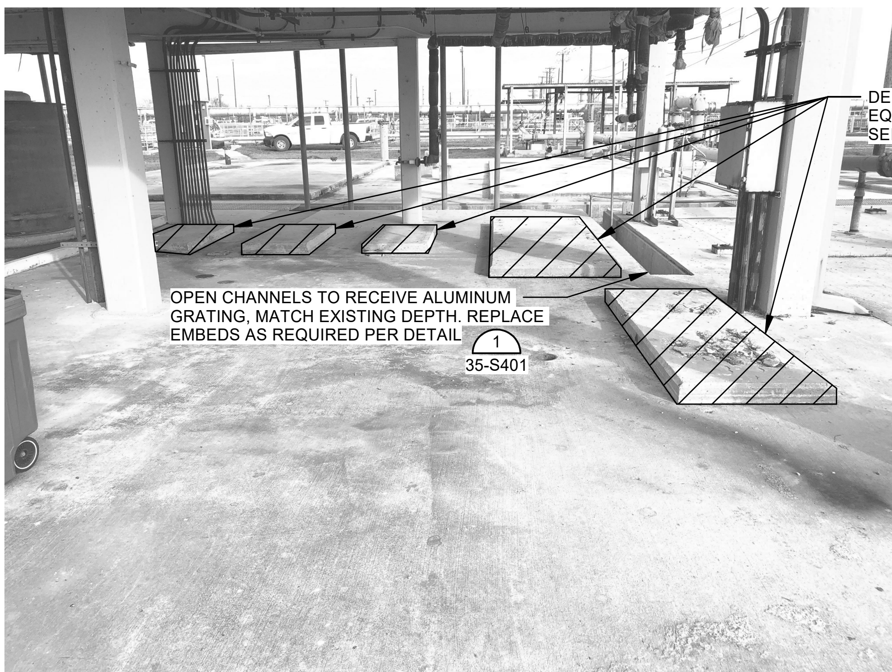
4 10-D123 VIEW OF EXISTING FACILITY LOOKING EAST SCALE: NONE
